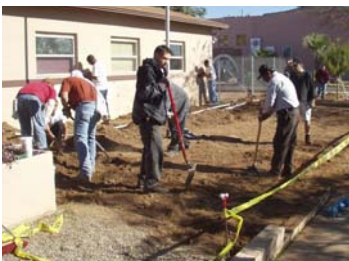
Laying the sprinkler system
