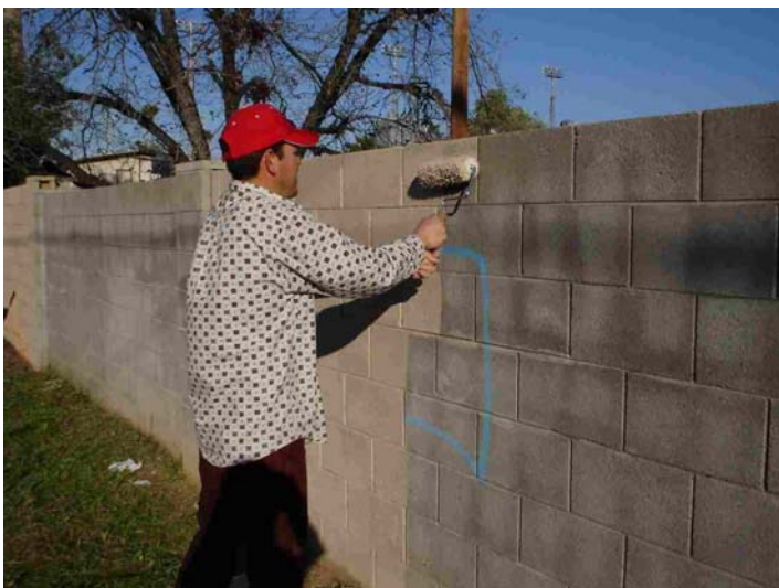
Jose putting the finishing touches!
